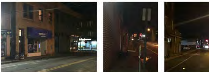
Example of Poorly Illuminated Streetscapes in Downtown Mineola
